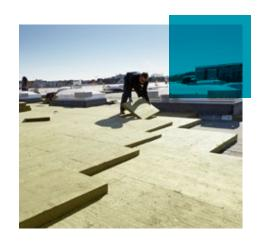
ROCKWOOL Toprock® fabricated stone wool insulation products are noncombustible – providing increased fire resistance, water resistant, and offer long-term dimensional stability. These components are engineered for compatibility with a variety of membrane types, air/vapor barriers, fasteners, and adhesives, making them critical components for a durable roof assembly in new construction and re-roofing.
